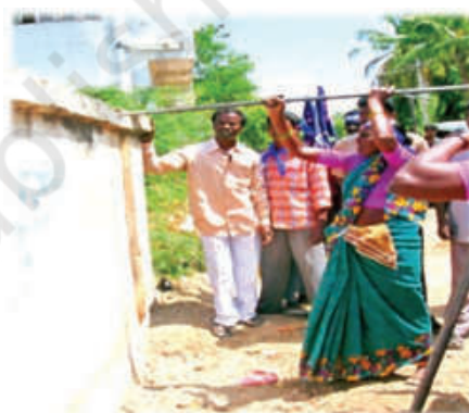
Members of the Safai Karamchari Andolan demolishing a dry latrine.
