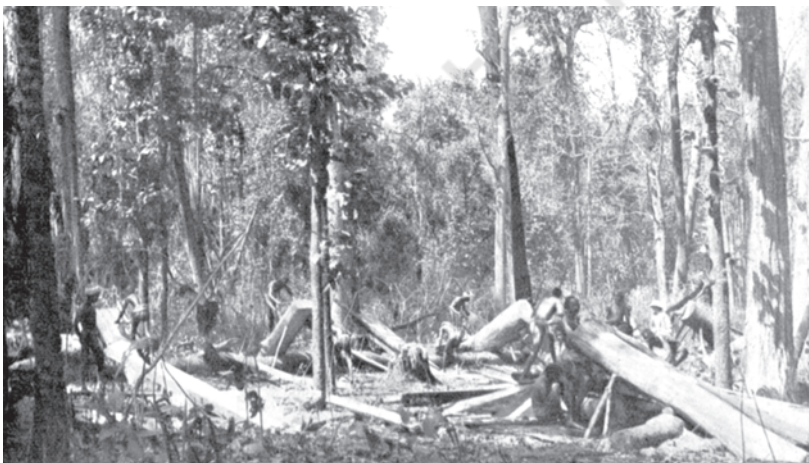
Fig.3 – Converting sal logs into sleepers in the Singbhum forests, Chhotanagpur, May 1897.
