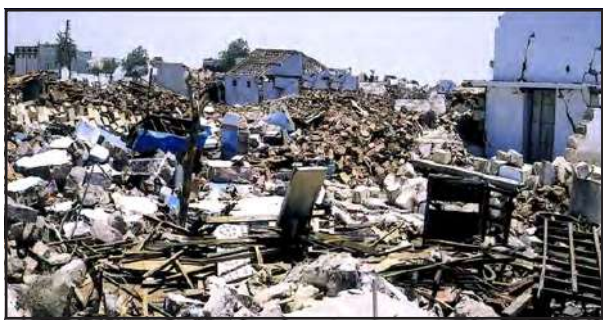
Figure 5.2 :The Bhuj earthquake 26 th January,2001
